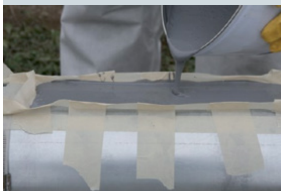
FIGURE 3: Polyurethane field joint coating (casting)
