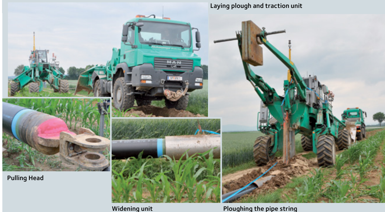
FIGURE 18: Laying of a water transportation pipeline using the plough technology
