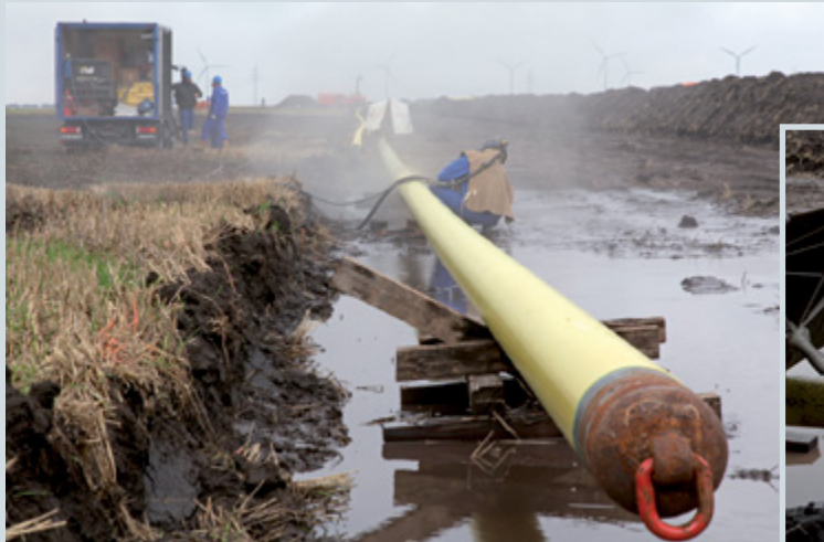
FIGURE 15: Field joint coating using a polyurethane resin
