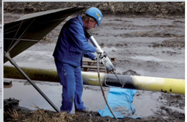
Field joint coating with polyurethane
