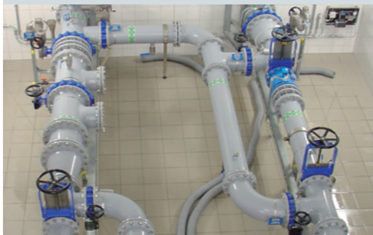
FIGURE 2: Polyamide-coated pipelines in a service station for drinking water
